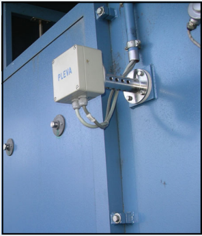
Fig. 2: FS 91 Exhaust Humidity Sensor
